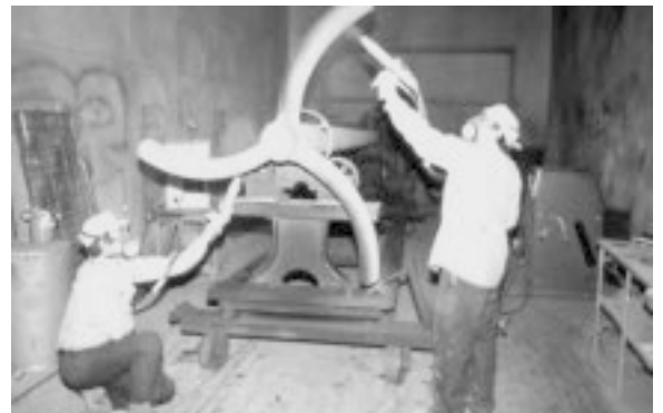
Figure 8.42 Electrostatic powder application of an agitator. (Courtesy General Plastics Corp.)
